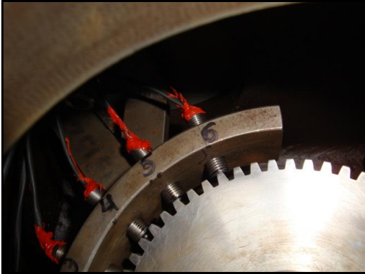
ECT's Mechanical Retrofit Using Magnetic Pickups, Brackets, and Speed Sensing Gear
