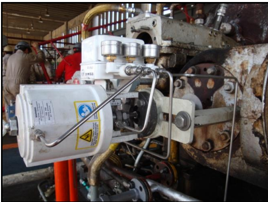
ECT's Mechanical Retrofit Using Pneumatic Actuator on the Steam Valve
