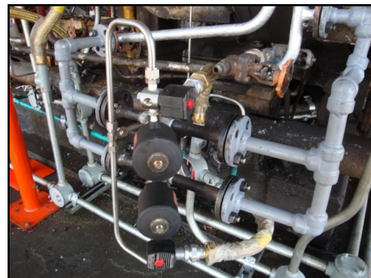
Redundant solenoid arrangement for trip & throttle valve
